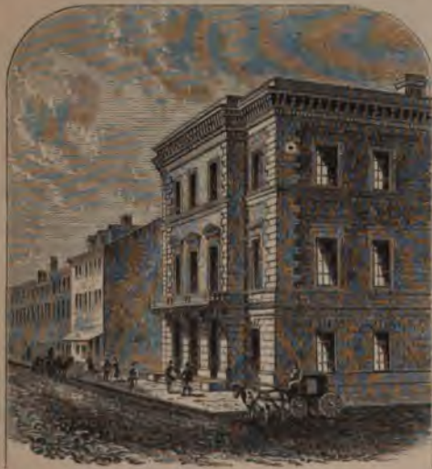
The Custom - House—Mobile, Alabama.
